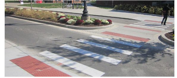
ADA accessible curb ramps with median
