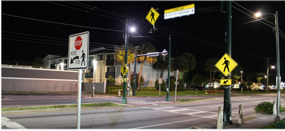
Crosswalk visibility improvements (Source: Florida DOT)
