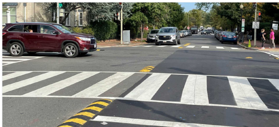
Curbing used for centerline hardening (Source: Minnesota DOT)
