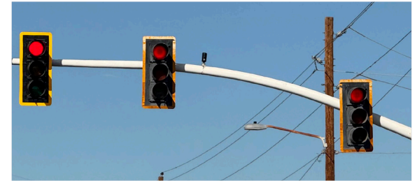
Reflective backplates on signal heads
