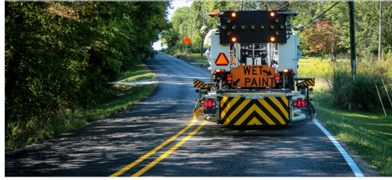
Striping improvements (Source: Indiana DOT)
