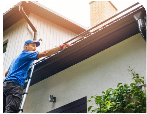
Clean gutters and downspouts in the spring and in the fall to ensure all debris is cleared out.
