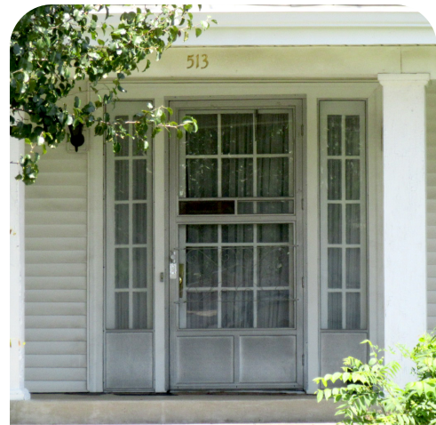
Add storm doors as a second full barrier against the elements (513 W. Main St.)
