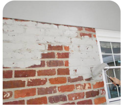
Do not paint masonry unless already painted or if the integrity has been damaged.
