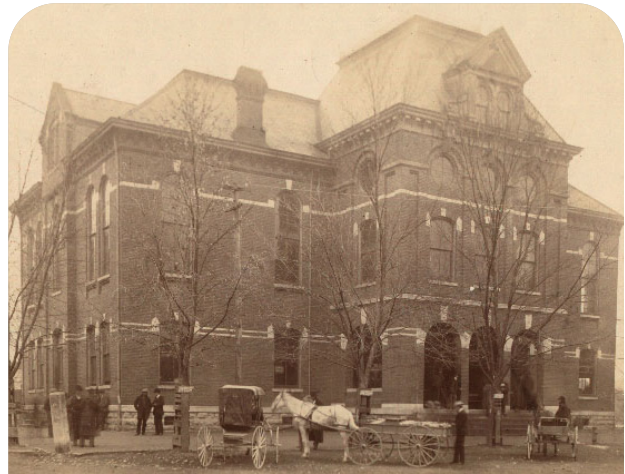
Wilson County Courthouse 1882. Courtesy: Tennessee State Library Archives, Image ID 5071
