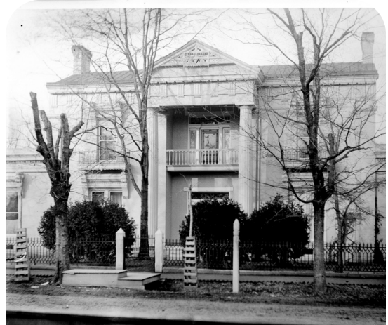
1828. Caruthers House, 241 W. Main Street. Courtesy Historic Lebanon.
