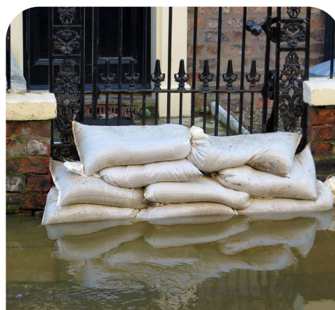
Utilize sandbags for flood protection and prevent potential water breaches.
