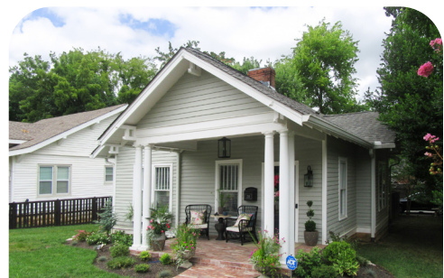
Preserve and avoid replacing sound wood material (211 E. Spring St.)
