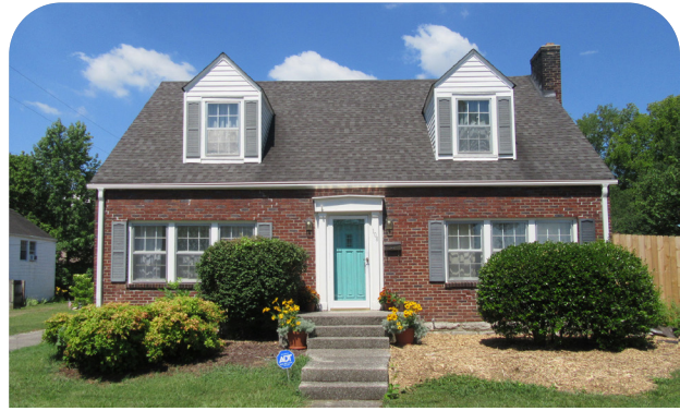
108 Pennsylvania Avenue, a c. 1933 Cape Cod, is a Contributing Resource within the Cumberland University Historic District
