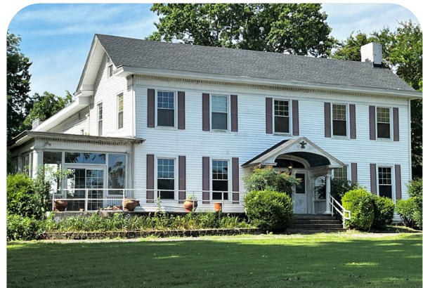
622 W. Main Street, c. 1911, is a Contributing Resource within the West Main Street Historic District.
