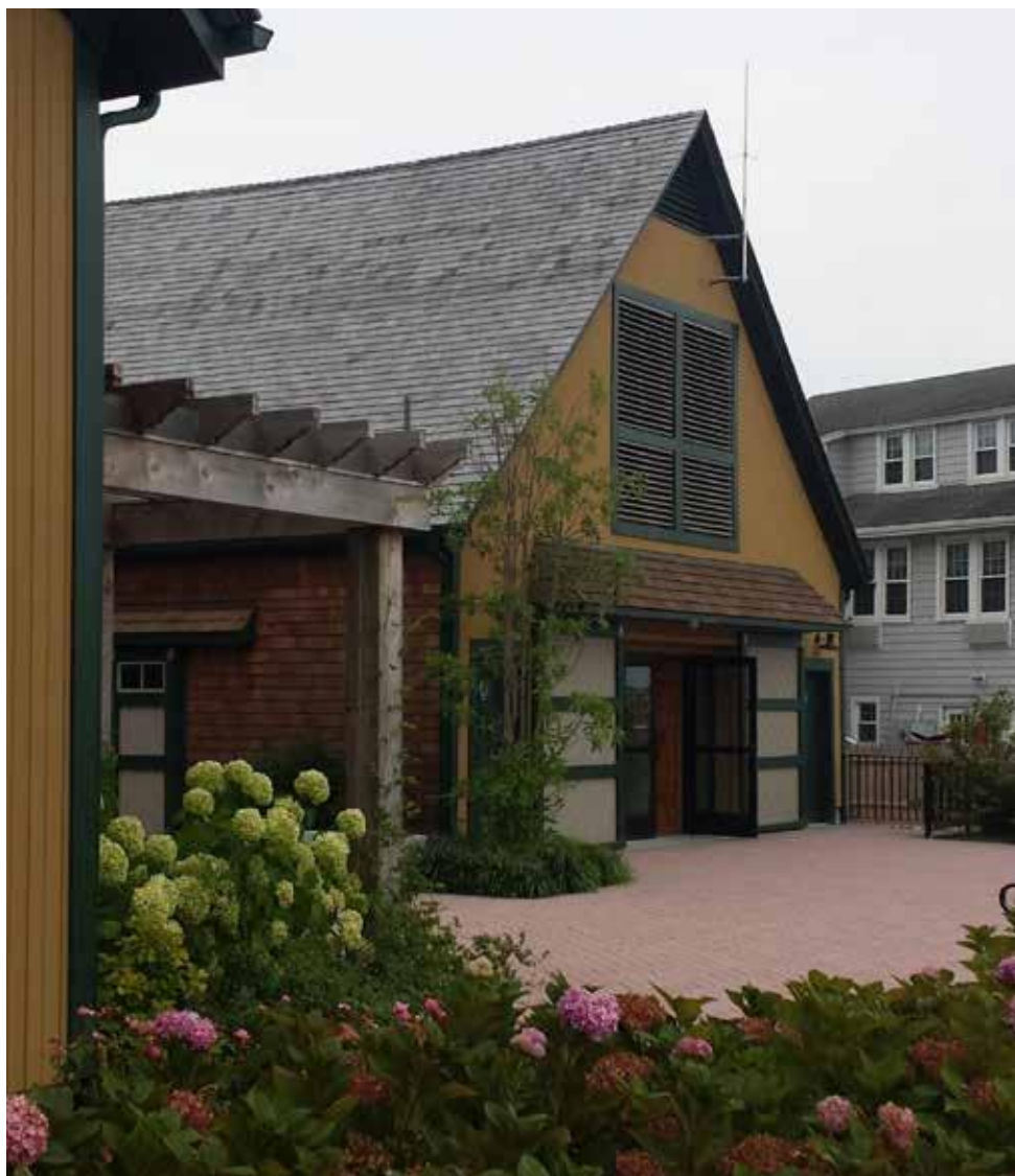
Figure 6: The mechanical room was relocated to the upper floor at the back of the building, discernible in this photo by the louvered vents. Photo: Jennifer Wellock/NPS
