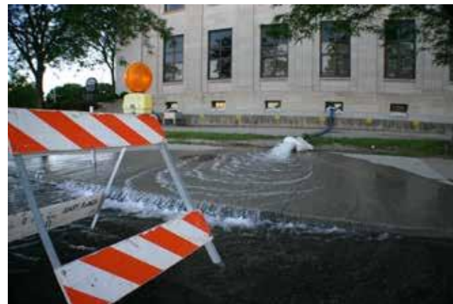
[65] Flood waters often must be actively pumped out of and away from the property, as seen in this image from Des Moines, IA. The pumping process should be designed to control the shift in hydrostatic pressure on the building and remove all flood waters that do not naturally drain or recede from the property. Photo: Chris Snider
