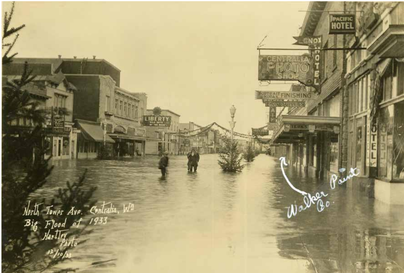
[4] As this 1933 image of North Tower Avenue in Centralia, WA, shows, flooding events have long been a major challenge for many communities. Photo: Lewis County Historical Museum
