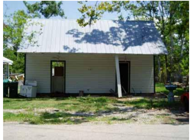
(a) Photo: Rubion Construction Co., LLC
