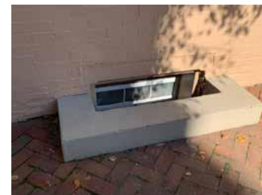
[55] A low flood wall or curb that is compatible with the historic character of the property can be constructed around basement windows to keep flood waters out. Photo: Jennifer Parker/NPS
