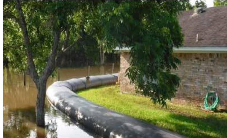
[21] A rural homeowner has deployed a water-filled temporary dam or water bladder to act as a floodwall around their residence. Water bladders require a storage area when not in use and the resources and time to fill them when a flood is imminent. Photo: Aqua Dam, Inc
