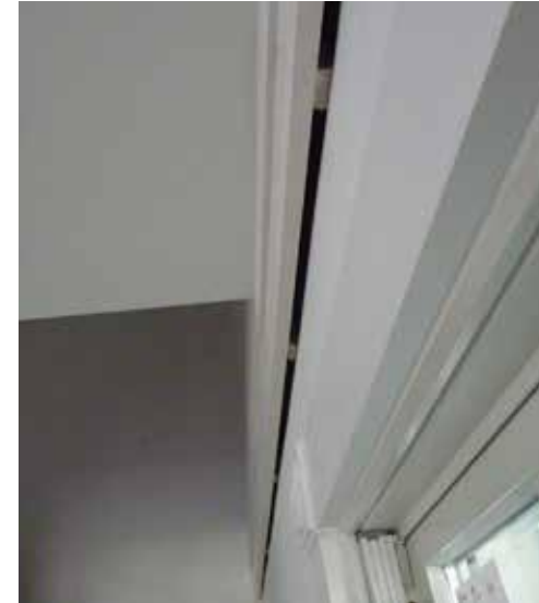
Figure 4: Crown molding covers an opening at the top of walls to allow air to circulate and dry wall cavities after a flood, seen here before the sacrificial insulating foam strip has been applied. Photo: Mary Delaney Krugman, JD, MSHP
