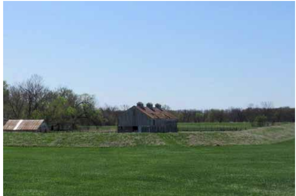
[31] This small-scale levee or berm has provided flood protection to this property in Chase County, KS, since the 1940s. Photo: Steve Samuelson
