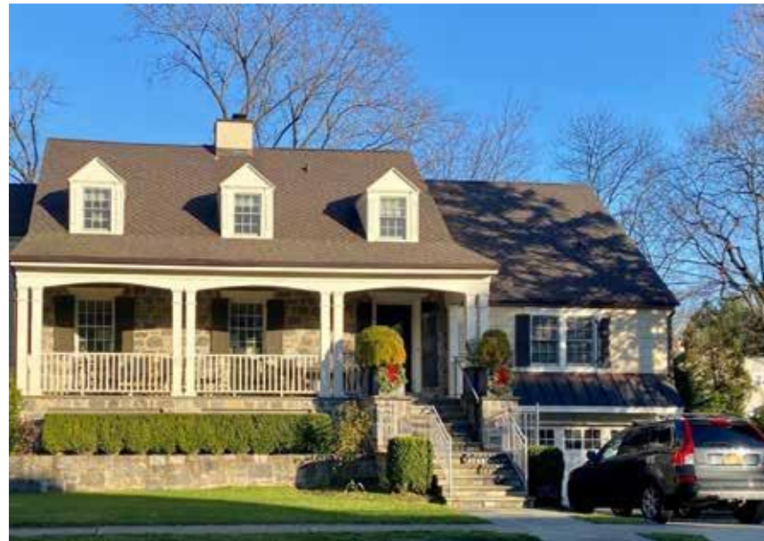
[93] This home has used elevated planting beds across the front of the house to bring the landscaping up higher and help screen the change in height. The stairs are stone, to blend in with the foundation and the planters, and a landing breaks up the long run of stairs at a point that aligns with the top of the planters. This provides a visual reference point for what was the original foundation height. The garage remains at grade level. Photo: FloodSavvy.com
