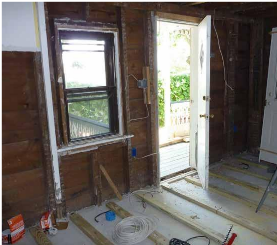
Figure 2: In-progress repairs after Hurricane Sandy. Walls are open to the interior for initial drying. A new concrete structural slab has been topped with treated wood sleepers in preparation for a new flood-damage resistant mahogany floor. Photo: Mary Delaney Krugman, JD, MSHP
