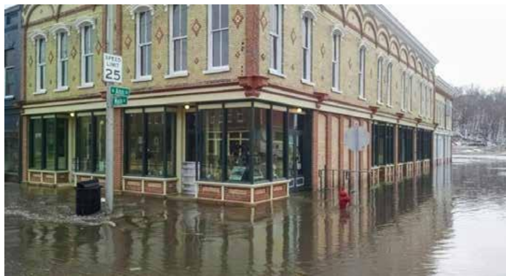
Figure 7: Floodproofing measures kept the water out of the Driver Opera House during a 2019 flood. Photo: Brian Mesmer
