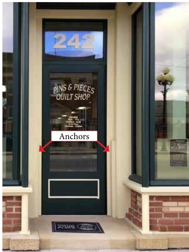
Figure 5: Door jambs were designed with integral anchors for attaching removable floodgates. The anchors are visible but painted to blend in. Photo: Heidi Brenum
