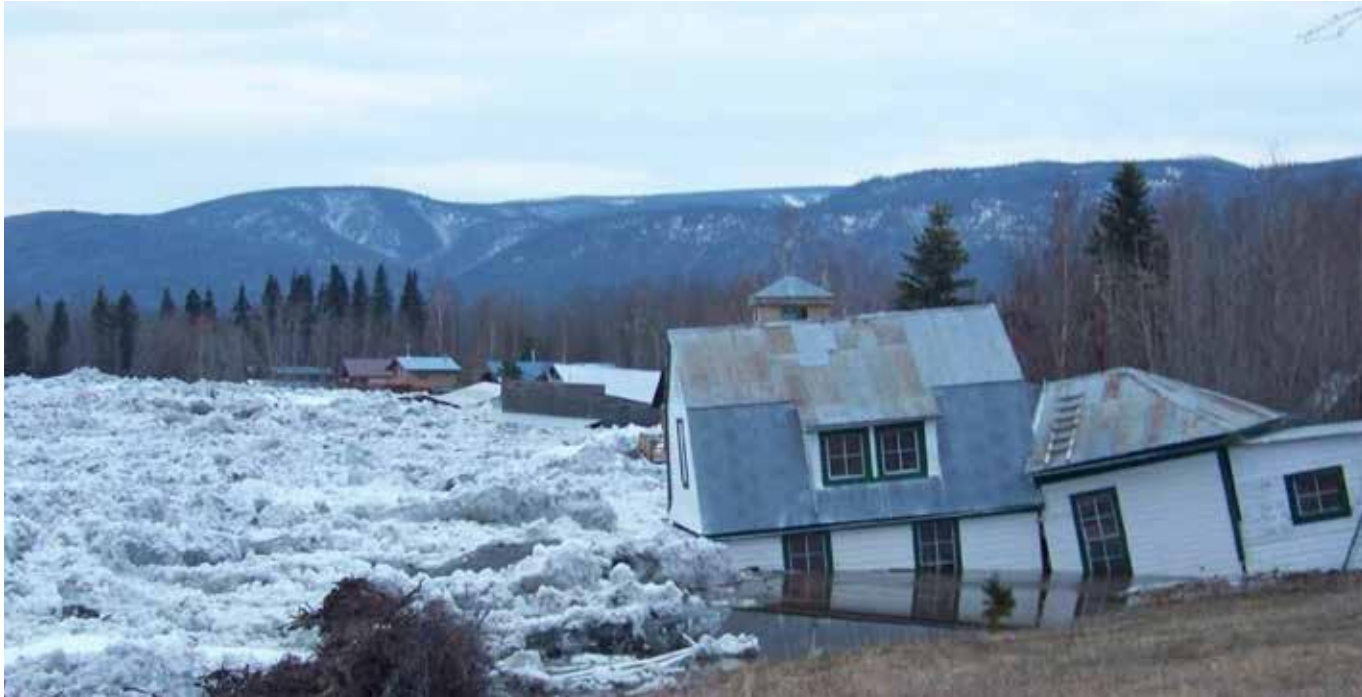
[5] In 2007 the Old Customs House located in the Yukon-Charley Rivers National Preserve, AK, was significantly damaged by riverine flooding. Historic properties that may not have flooded before are increasingly affected by larger flood events. Photo: Carl Stapler/NPS
