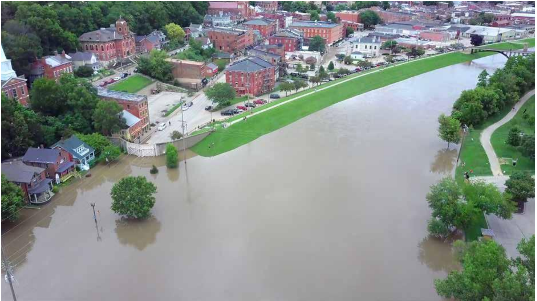
[19] Community-scale interventions, such as this combination of a flood wall, levee, and floodgates in Galena, IL, can protect multiple historic resources and maintain the character and integrity of entire historic districts and neighborhoods. Photo: GalenaGuide.com
