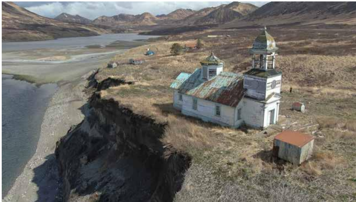
[13] The Church of Our Lord Chapel, Karluk, AK, was built in 1888 and is the oldest Russian Orthodox Church in Alaska. In danger of collapse into the Karluk River, the erosion of the bluff has been rapidly escalating, and the church sits only 25 feet from the edge. The vulnerability of the property at the edge of a river requires frequent monitoring, but a more long-term solution will be necessary for the continued preservation of the building. Photo: Tom Pillifant
