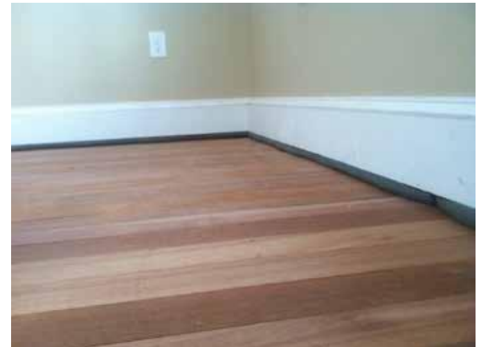
Figure 5: Mahogany wood floor and baseboard with a gap at the base for future venting. Foam insulation strip fills the gap and will be covered with removable trim. Photo: Mary Delaney Krugman, JD, MSHP
