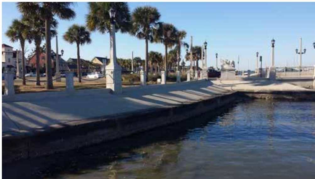
[34] Some flood protection structures are historic, such as this seawall in St. Augustine, FL. The seawall was constructed in sections over time beginning in 1696 near the Castillo de San Marcos. Photo: Jennifer Wellock/NPS
