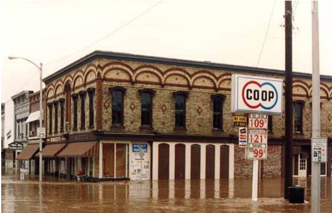
Figure 1: This 1993 flood was one of several events that led to the listing of the Main Street Historic District in the National Register. Photo: Lafayette County Historical Society
