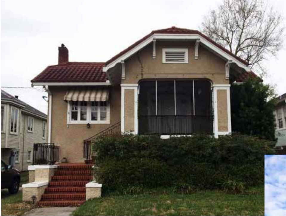
(a) Photo: Rubion Construction Co., LLC
