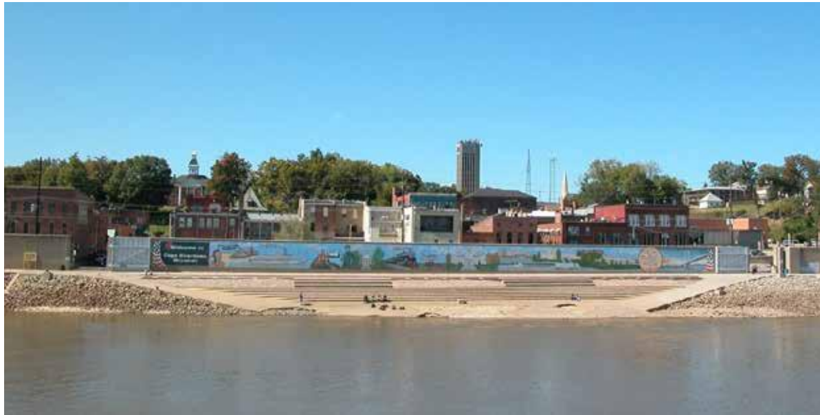
[33] A large floodwall protects the historic downtown of Cape Girardeau, MO, from the Mississippi River. Photo: VisitCape
