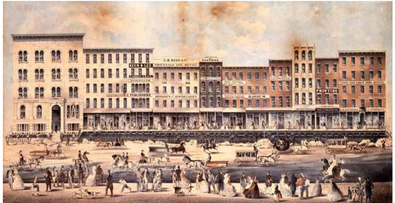
[74] Elevating masonry buildings built to the side lot lines can be difficult but has been done historically. This illustration shows an entire merchant block in Chicago being elevated at one time in 1857, as part of a larger plan to elevate the entire downtown area by four feet. Photo: Chicago History Museum, ICHI-059709
