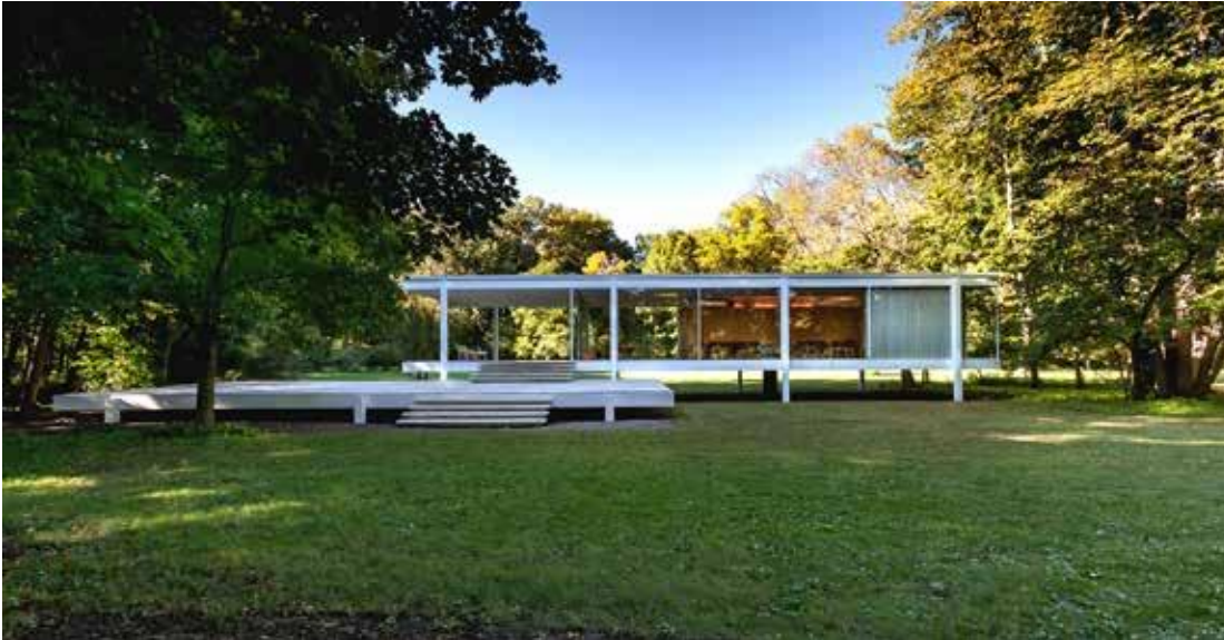
(a) Photo: Mike Crews Photography
