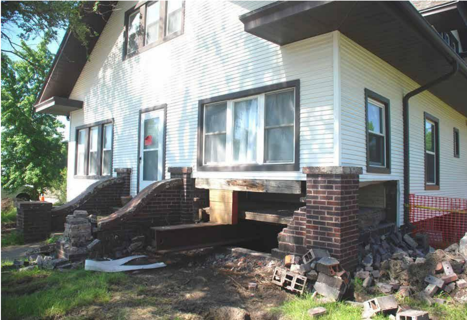
[72] Filling a basement requires access to bring the fill below grade and to maneuver compacting equipment in the space. In this example, a prior flood-damaged section of the foundation wall created an opening that allowed earthmoving equipment access to the basement. The exterior will be repaired once work is complete below grade. Photo: Mitch Paine
