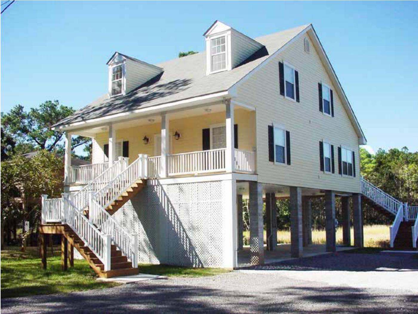
[82] Little can be done to mask or alter the appearance of a tall foundation. Once a building has been elevated the equivalent of a story or more, the overall proportions and scale of the building is often changed, resulting in diminished historic character. Photo: Courtesy of the Southern Forest Products Association
