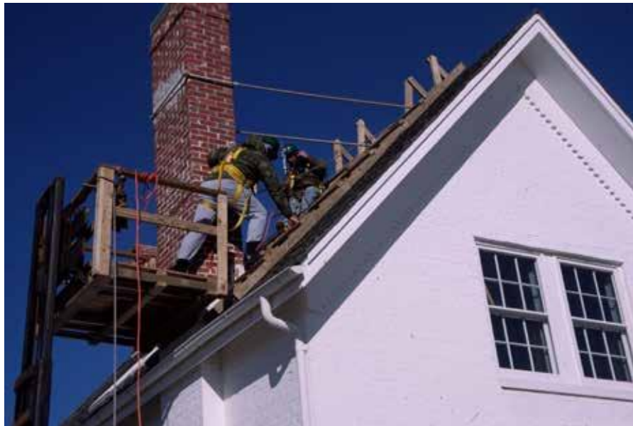
[113] Fragile features like chimneys should be evaluated and braced before a building is moved. Photo: Mike Booher/NPS
