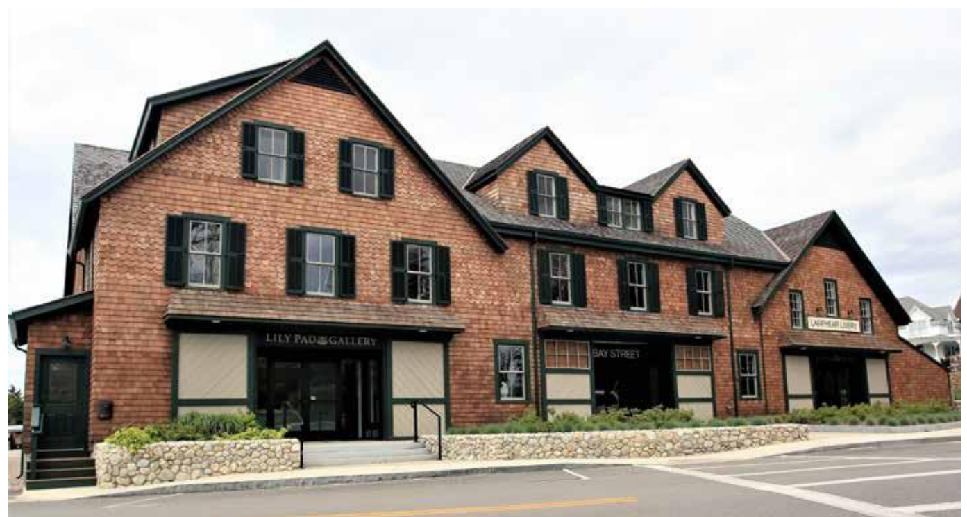
Figure 5: View of the building after the floodproofing and rehabilitation project was complete. The historic barn doors and many historic windows were preserved. Damaged or missing shingle siding was replaced in kind. The foundation is now two feet taller than it was at the start of the project. Wet floodproofing of the first floor provides additional resiliency and protection for floods that exceed the new elevation height. Photo: Pariseault Builders
