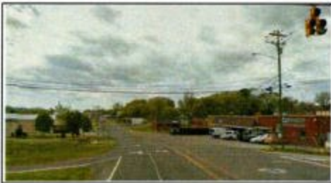
Existing non-descript intersection at Carthage Highway
