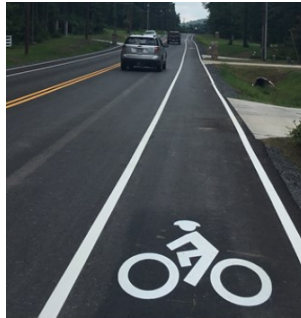
Figure 3: Narrowing travel lanes for motorists with bike lane markings
