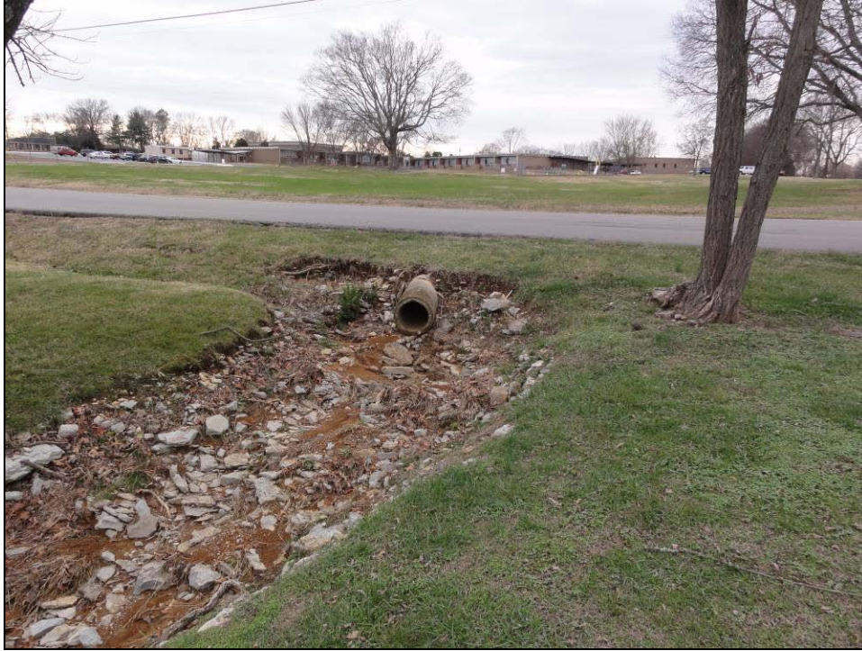
Item 5 – Mayfair Dr. between Sam Houston Dr. and Lealand Ave. Repair end of 18” RCP and install erosion control measures. Picture 1827.
