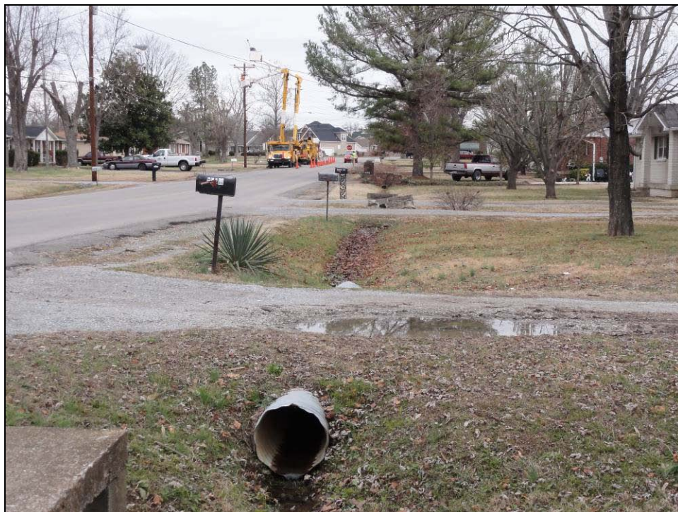
Item 2 – 418 Oakdale Dr. Clear debris from driveway culvert (shown in background). Picture 1796.
