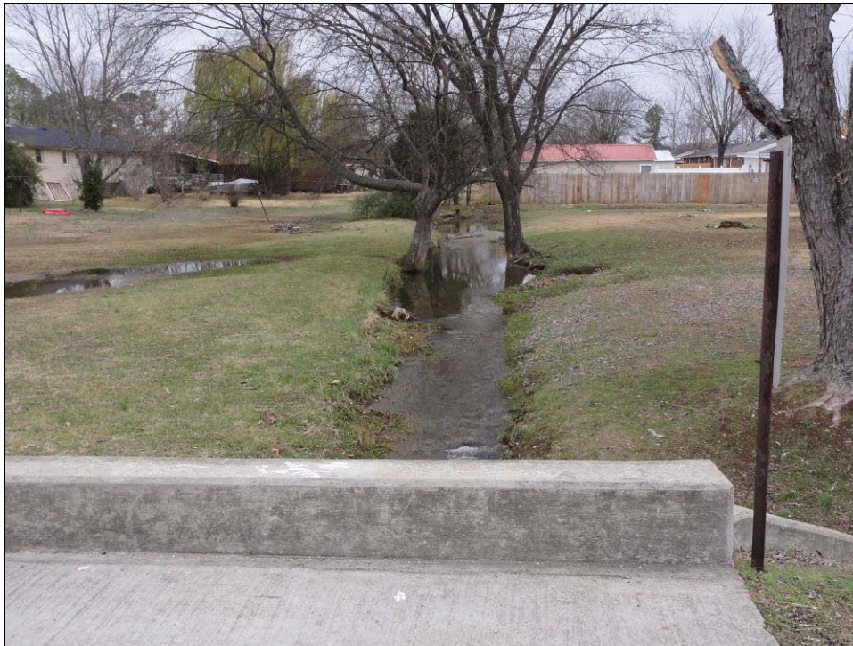
Looking east from Marks Cir. Picture 1812.
