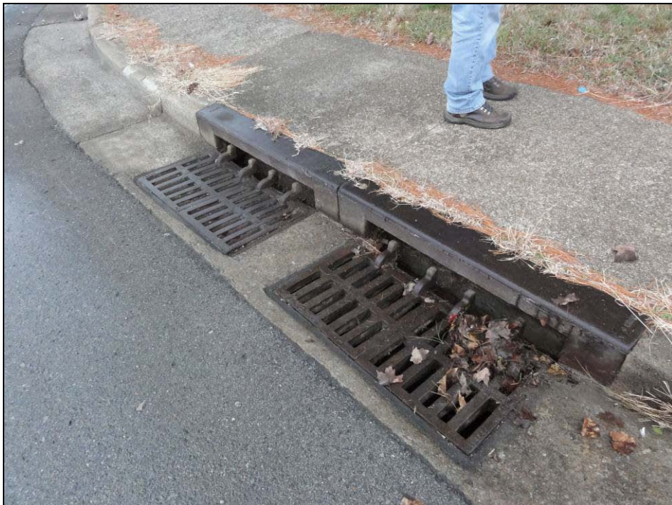
Item 16 – W. Main St. and S. Hatton Ave. Clean debris from catch basin grate. Picture 2217.
