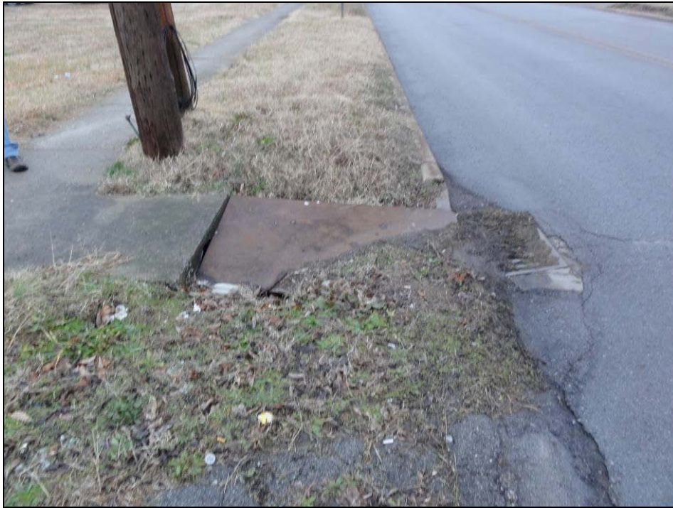
Catch basin cover and grate. Picture 2256.
