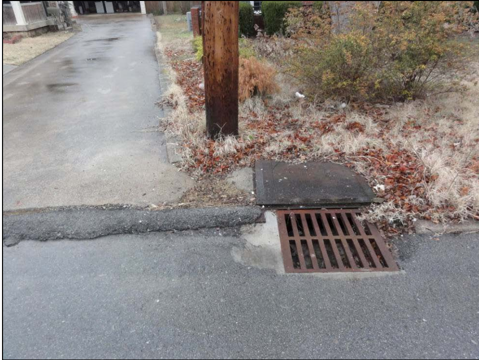
Item 13 – 217 Cumberland Dr. Clean debris and sediment from under catch basin grate. Picture 2197.
