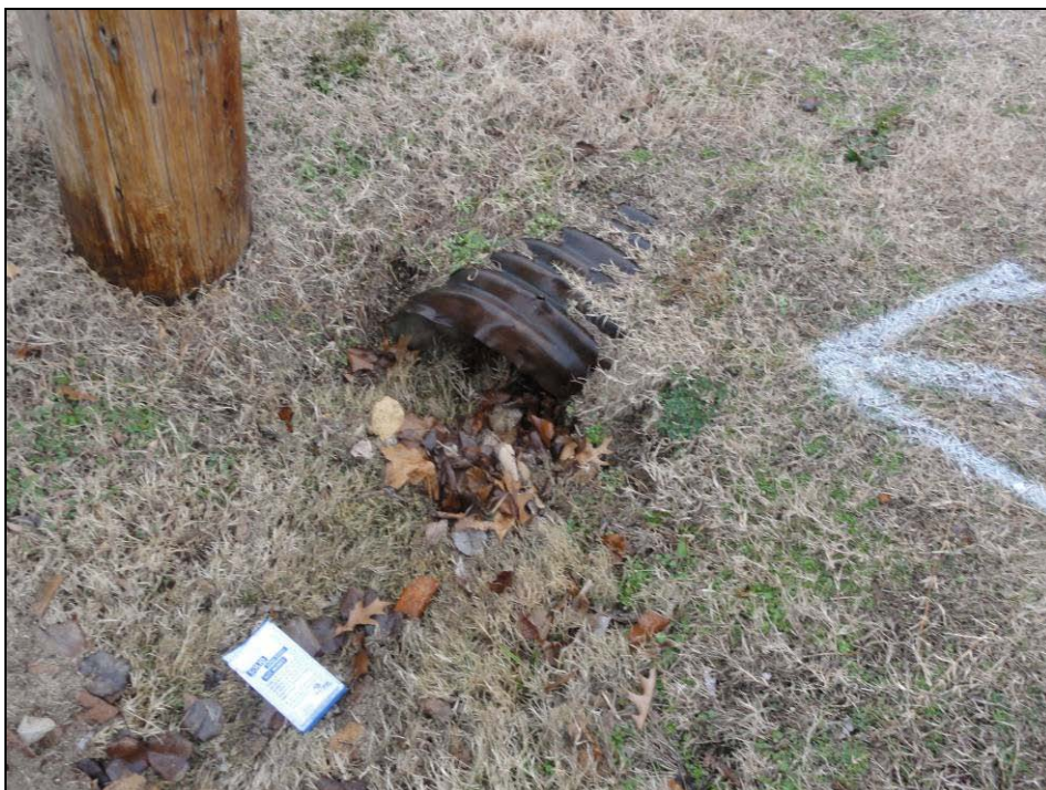
Item 6 – West side of S. Greenwood St. just south of University Ave. Clear sediment and debris from 12" CMP. Picture 2177.
