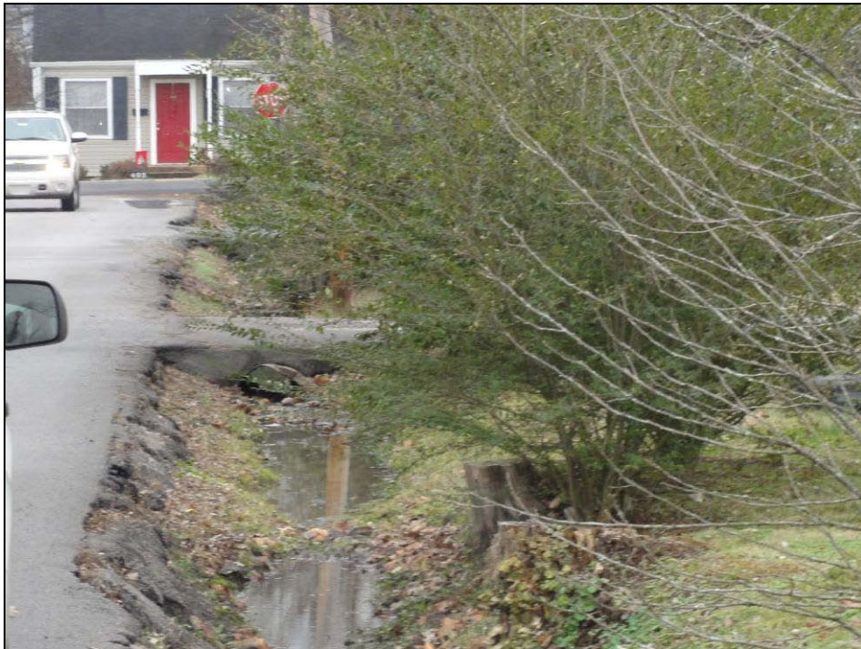
Ditch & driveway culverts on the north side of Martin Ave. Looking east. Picture 2364.
