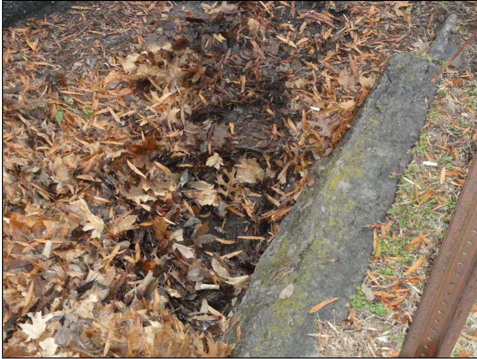
Item 17 – W. Spring St. and S. Tarver Ave. Clean debris from culvert inlet. Picture 2223.
