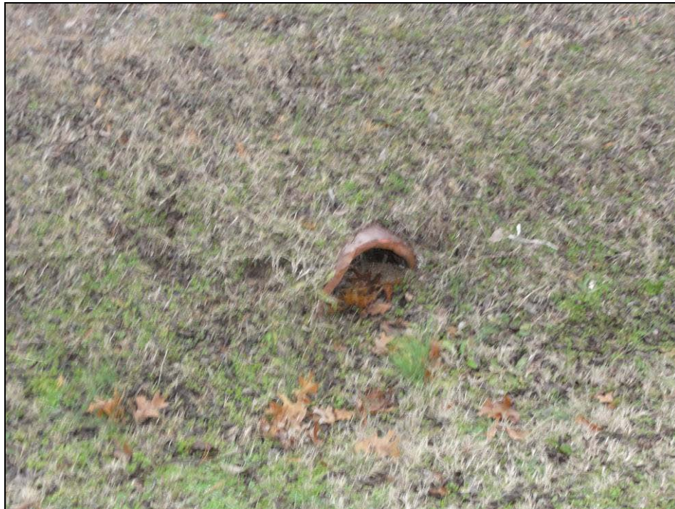
Item 29 – 224 S. Tarver Ave. Flush sediment and debris from 12” clay pipe. Picture 2304.
