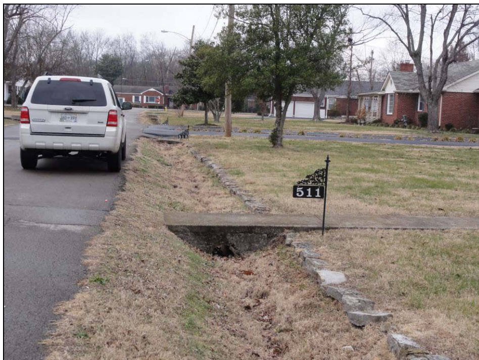
Looking west towards Pennsylvania Ave. Picture 2383.
