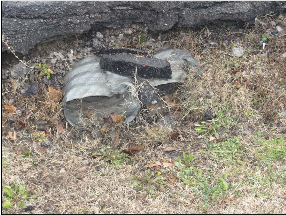
Inlets of 2 – 14” x 10” ellip. CMP’s. Picture 2184.
