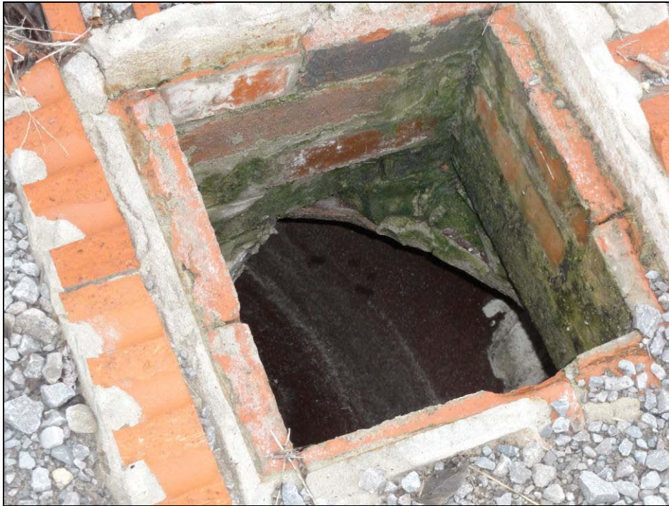
Item 27 – 319 S. Maple St. Install grate on catch basin. Picture 2272.
