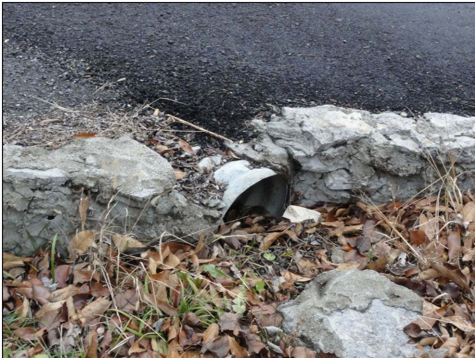
Item 38 - Martin Ave. and Cleveland Ave. Clear debris from ends of 10” CMP. Picture 2342.
