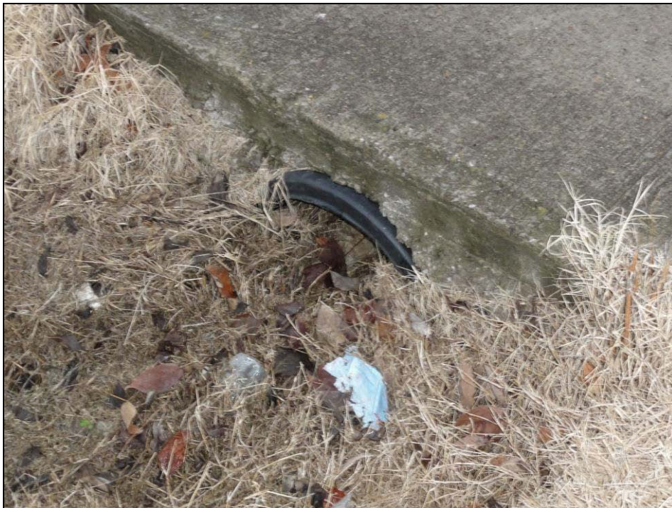
HDPE Inlet. Picture 2255.
