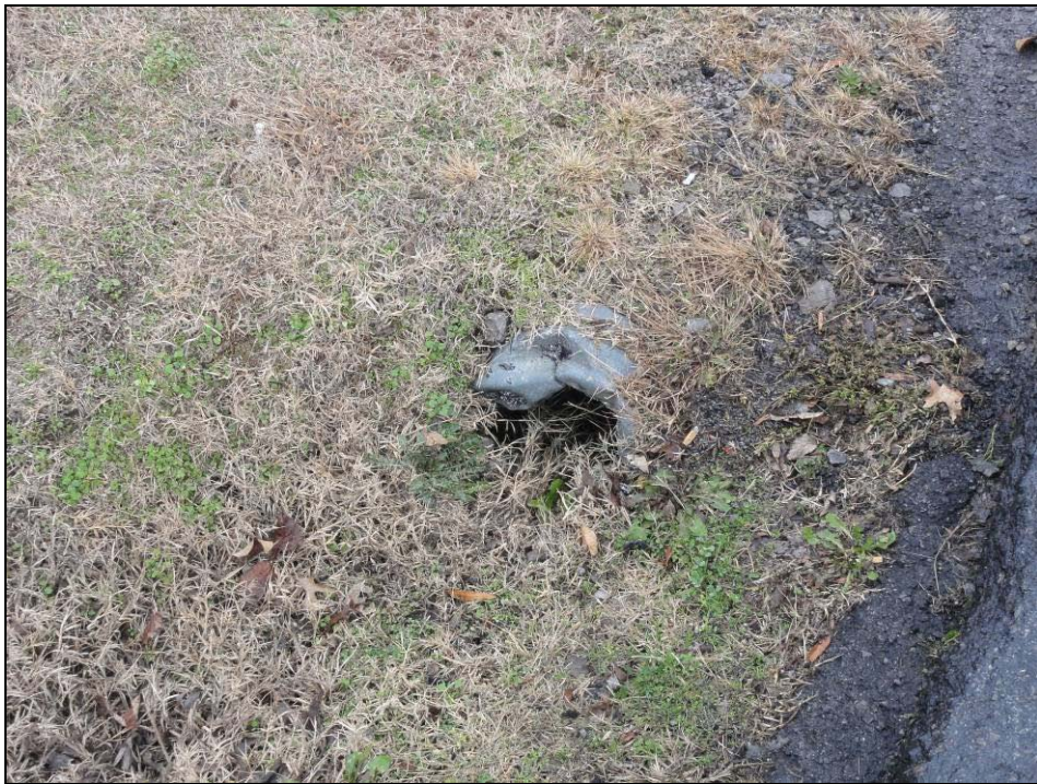
Item 8 – West side of S. Greenwood St. north of McClain Ave. Repair pipe end section, clear sediment and debris from CMP. Picture 2182.
