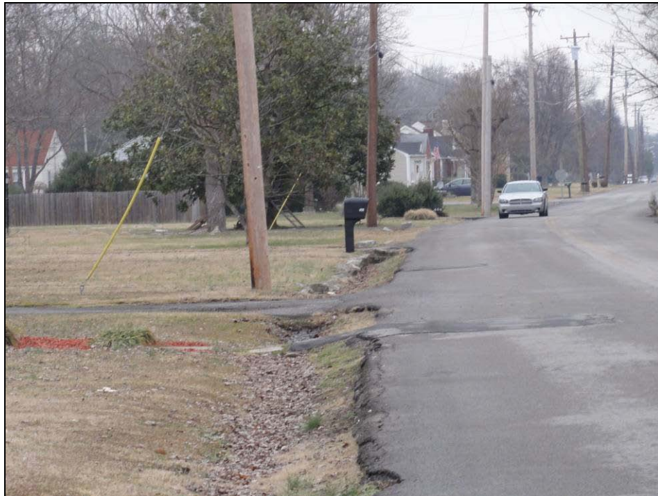
Item 48 – Pennsylvania Ave from Leeville Pk. to Martin Ave. View is looking north from 410 Pennsylvania Ave. Clear debris and sediment from road side ditch and culverts on the west side of Pennsylvania Ave. Approx. 900 LF. Picture 2390.
