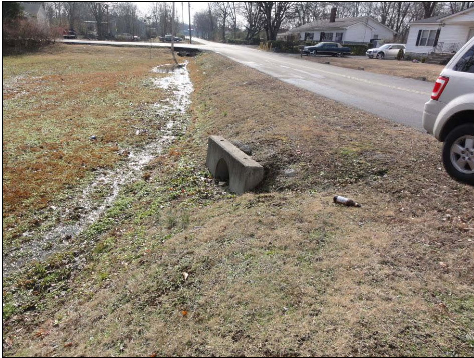
Item 52 – Leeville Pk. and Cleveland St. Clear sediment from 15” RCP. Picture 2430.
