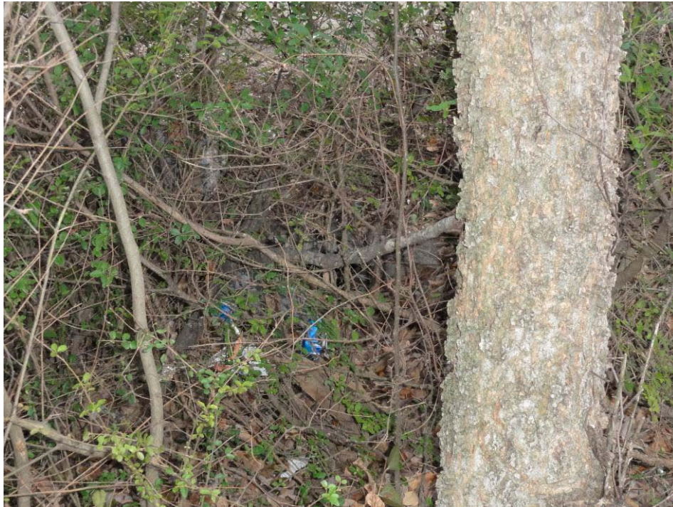
Item 25 – 316 S. Maple St. Clear brush and debris from pipe opening. Picture 2268.
