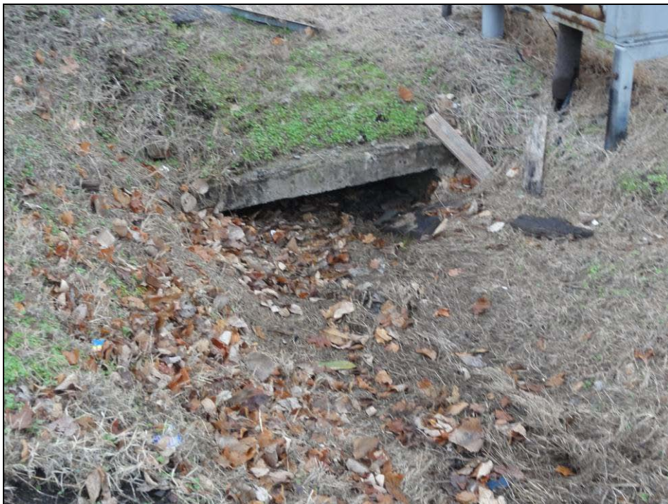
Item 14 – W. Main St. and railroad. Clean sediment and debris from opening of 4' x 2' box culvert. Picture 2213.
