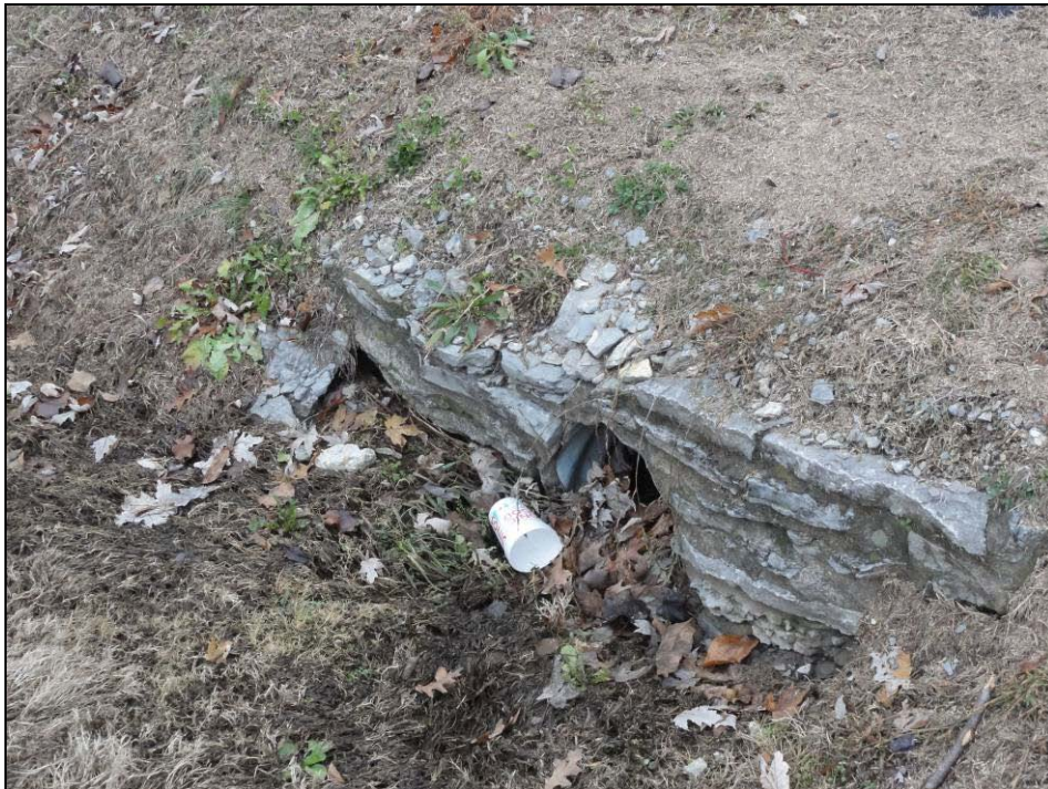
Item 32 – S. Tarver Ave. north of St. Frances Cabrini Catholic Church. Clear debris and sediment from both ends of 12" CMP. Picture 2312.
