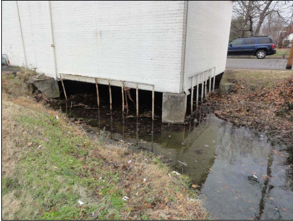
Looking north the rear of 502 W. Main St. Picture 2278. Bridge inlet is under building. Note bridge abutment footing on right side of photo.
