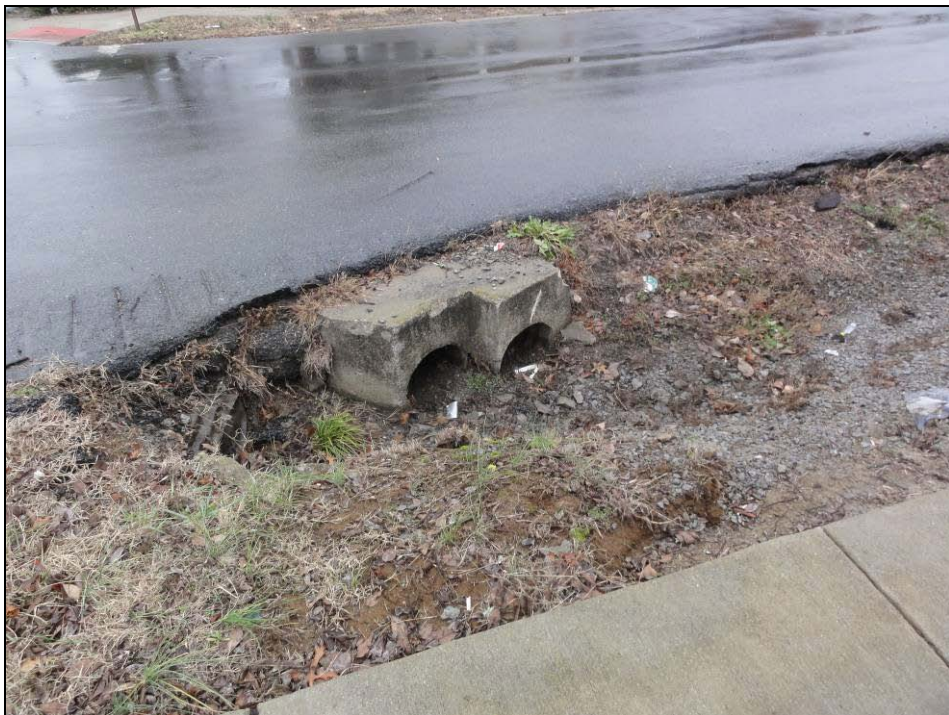
Outlets of 2 – 14” x 10” ellip. CMP’s. Picture 2189.
