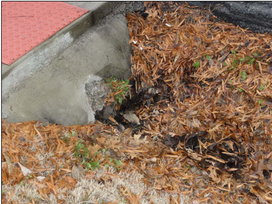
Item 18 – W. Spring St. and S. Tarver Ave. Clean debris from culvert inlet. Picture 2224.
