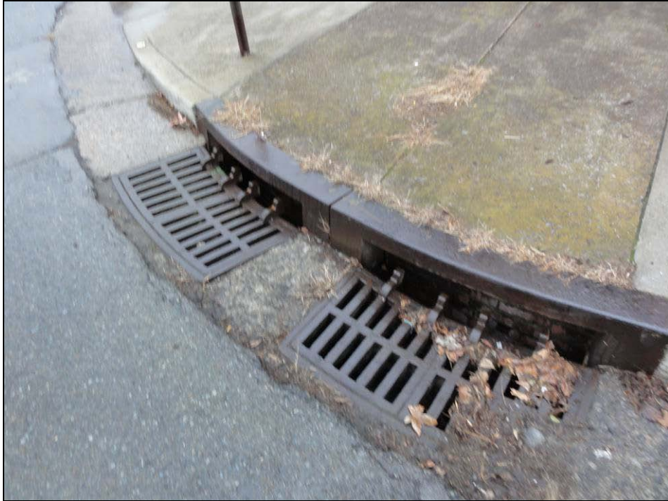
Item 15 – W. Main St. and S. Hatton Ave. Clean debris from catch basin grate. Picture 2215.
