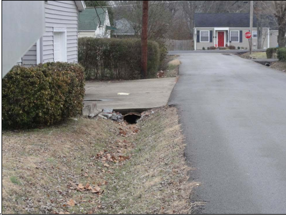
Ditch & driveway culverts on the south side of Martin Ave. Looking east. Picture 2363.
