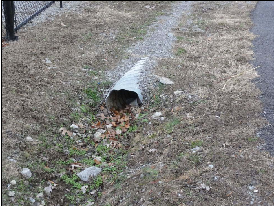
Item 31 – East side of S. Tarver Ave. north of St. Frances Cabrini Catholic Church. Clear debris from 12" CMP. Picture 2311.
