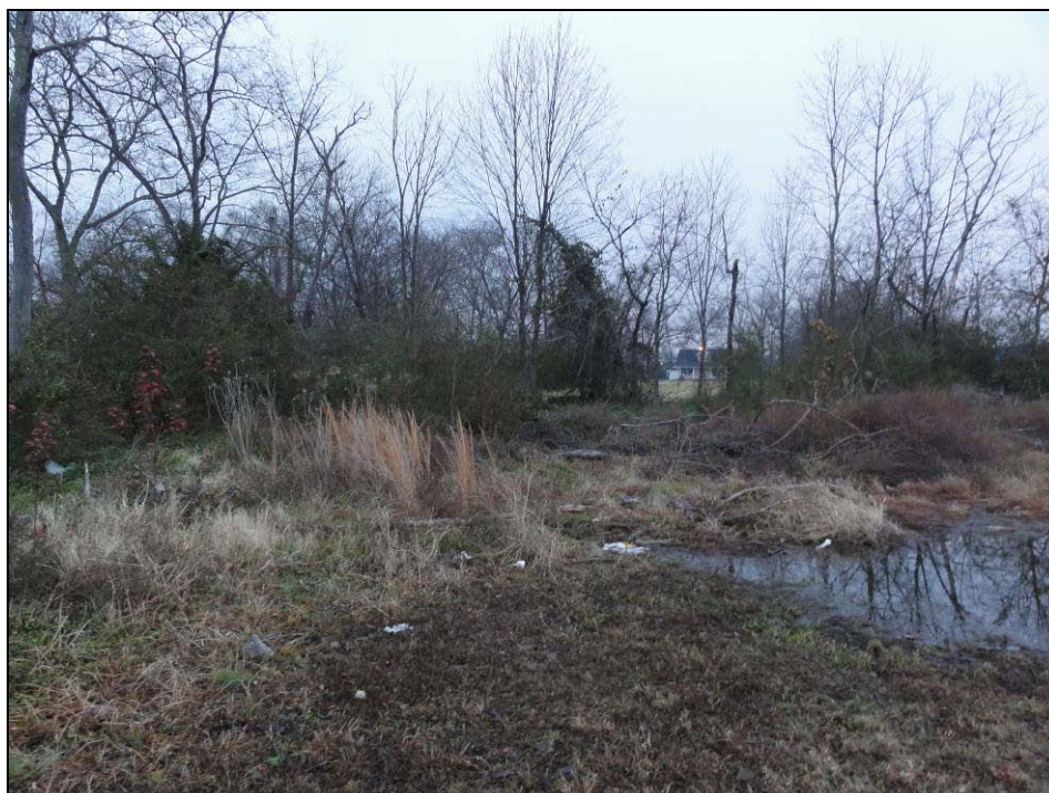
Looking east toward former detention pond and concrete riser structure that is filled in with dirt. Picture 2251.
