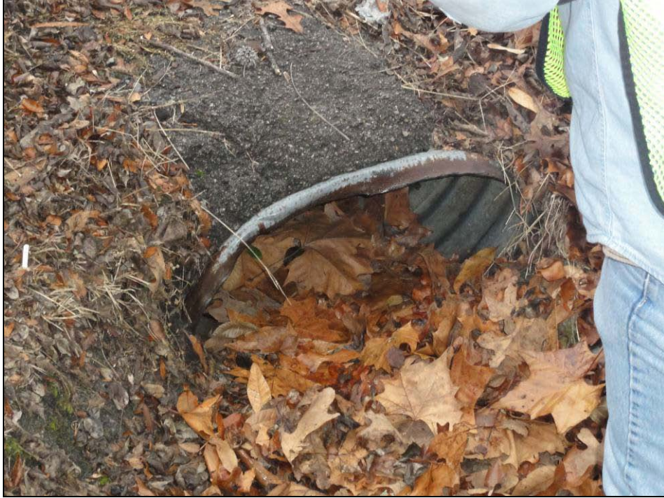
Item 21 – W. Sprint St. and Pennsylvania Ave. Clean debris from 20” x 14” ellip. CMP. Picture 2234.
