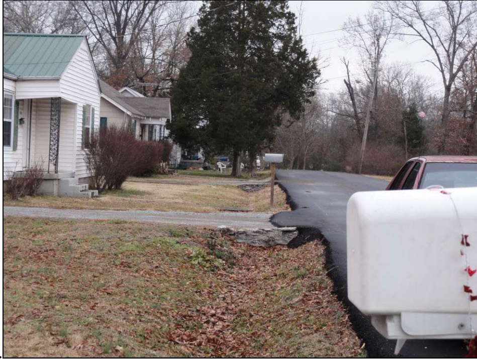
Item 39 – Cleveland Ave north of McClain Ave, looking north. Clear debris and sediment from driveway culverts and ditch. Approx. 400 LF Picture 2344.
