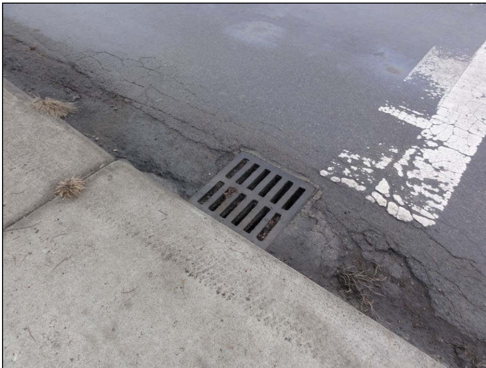
Item 4 – S Greenwood St. at W. Spring St. Clean catch basin grate. Picture 2173.
