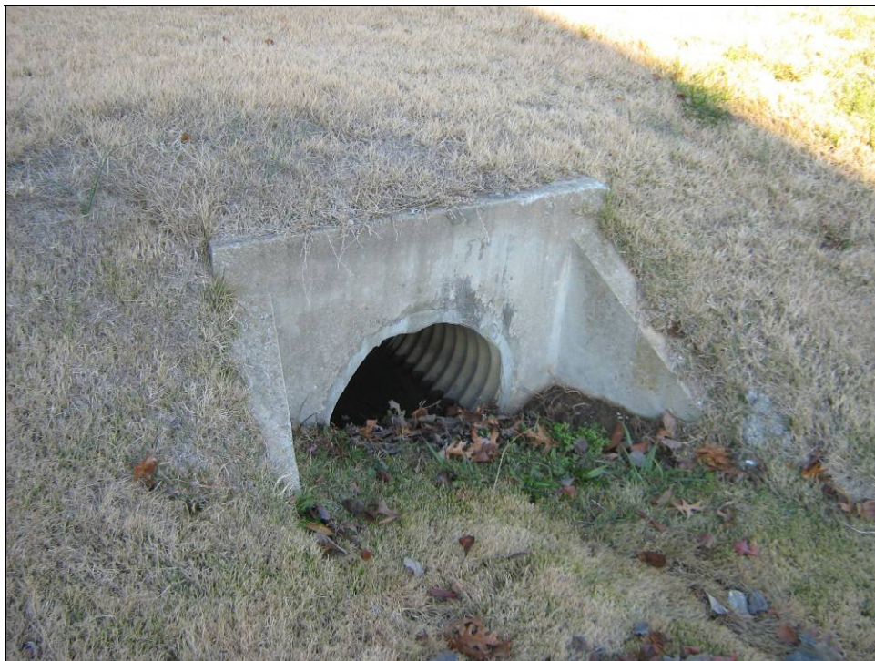
Item 6 - Lexington Dr. north of Antietam Dr. Clean silt from 36" CMP outlet. Picture 2368.
