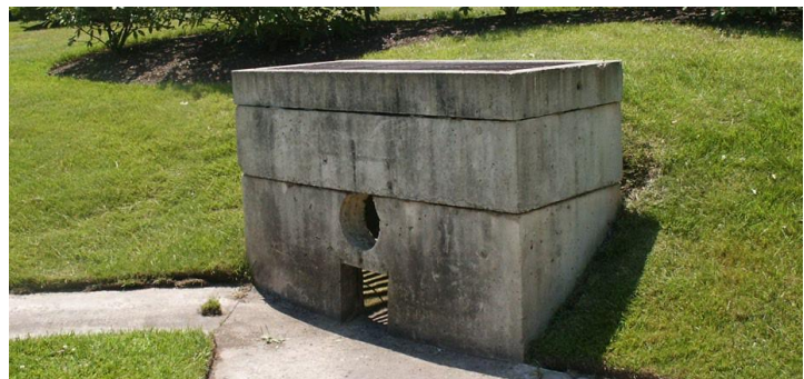
Figure 2: A typical outlet structure
